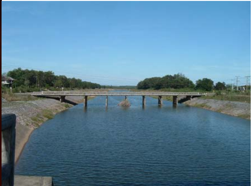
Irrigation projects to solve flooding problem
