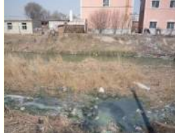
Sewage (under construction) China
