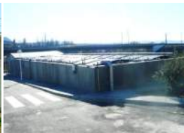
Public sewage Spain
