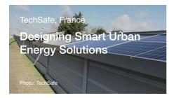
"SunScreen" is a road-side wall that acts as an extremely effective noise barrier and generates solar power. With aesthetics a major concern surrounding most renewable energy technologies, TechSafe had to ensure that SunScreen could easily blend into its surroundings. The solution: a simple and clean design, with a neutral and muted earth-tone color palette.
